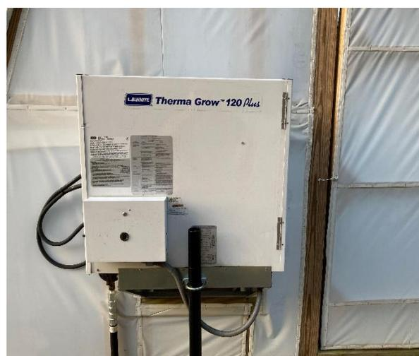
**Figure 22.** (left) Covering greenhouses with 50% opacity plastic for winter protection, and (right) outdoor mounted, direct fire, forced air heat for high efficiency heating.
