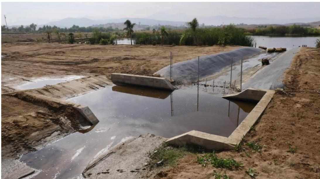
**Figure 3.** Sediment forebay designed for easy clean out.
